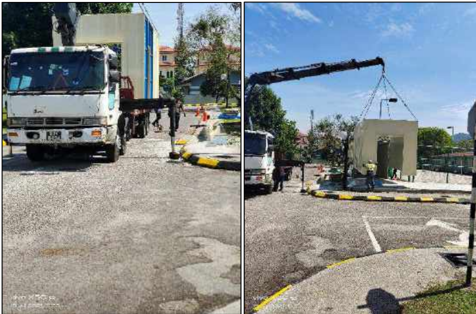
Figure 4.3.4.4: Relocation of modular laboratory in NPHL
